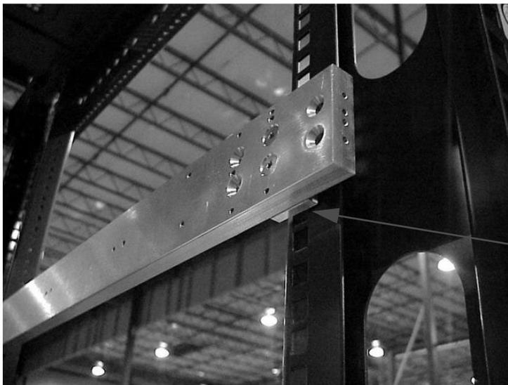
For the right rail mount, a spacer block is required to maintain the correct spacing for the rail mount in the rack (Two per rail mount).
